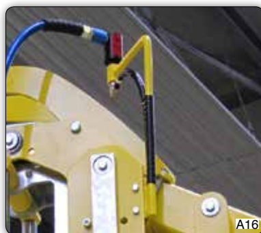
Top compressed-air feed.
